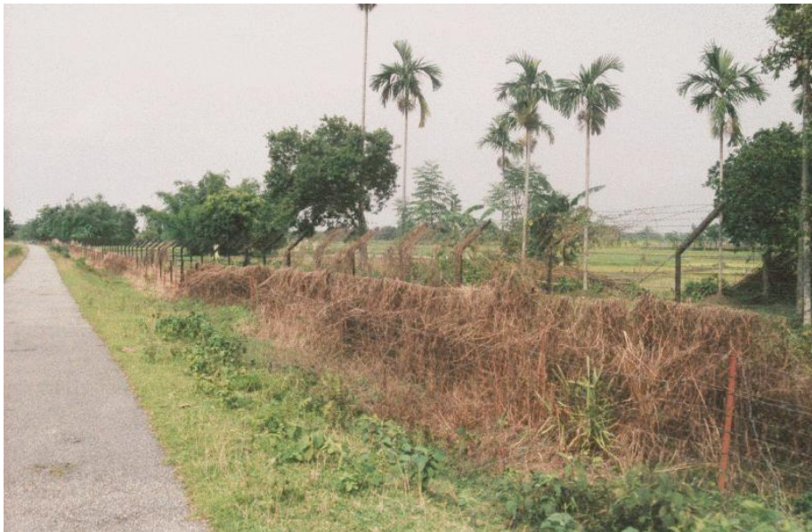
Photo 8. Border fence and road, Haldibari-Chilahati border crossing.
