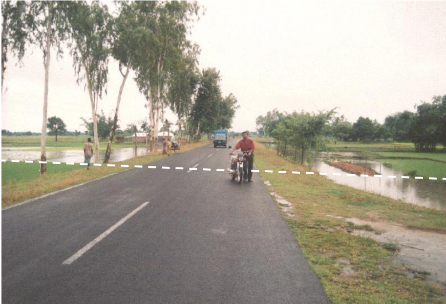
Photo 17. Bangladesh National highway traversing Indian Putimari enclave #59/18. Looking south into enclave from Bangladesh. Note absence of any signs or break in tarseal that would indicate the boundary. Compare Fig. 7b.
